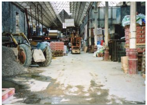
Building supplies under the Station roof
